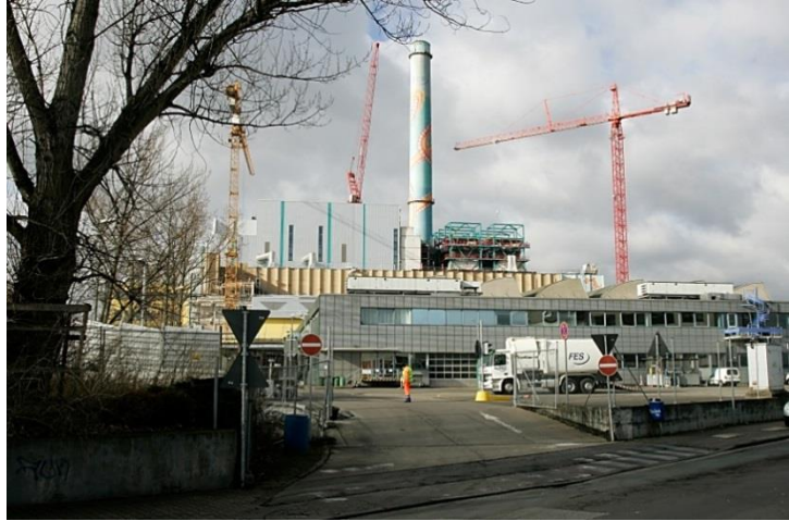
Waste incinerator in the North of Frankfurt
